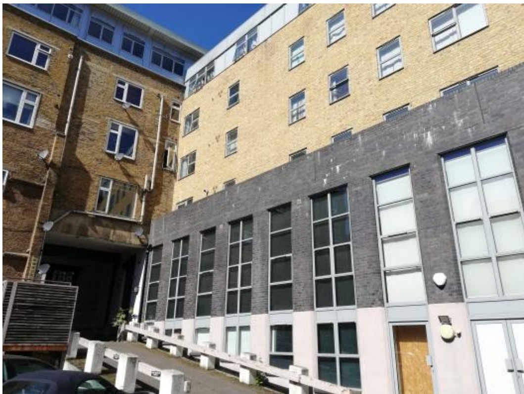
22 Calvert Avenue premises and access ramp
