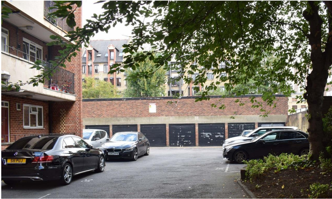
Figure 2: The garages to be demolished.
