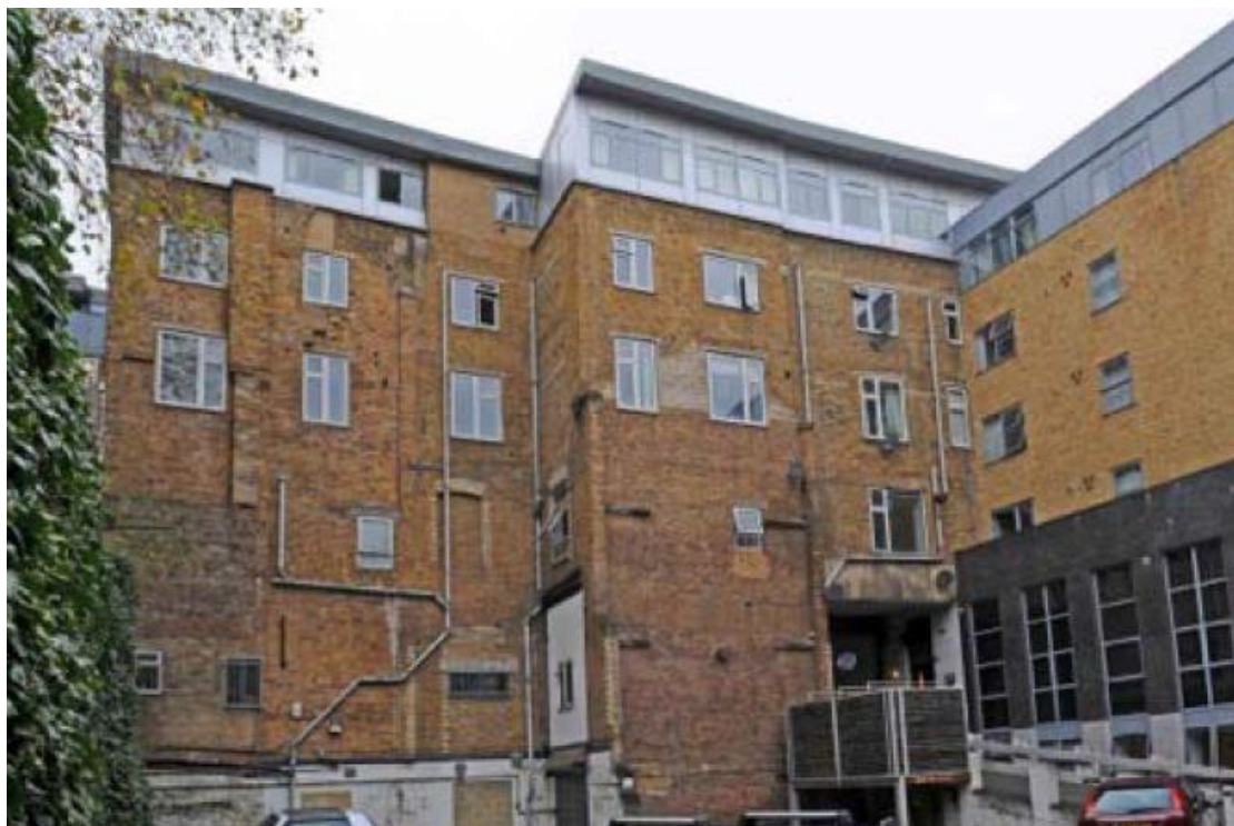
Rear of Walker House from car park
